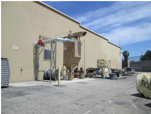
Figure 6: Dust collector on southwest elevation, view looking northeast (GPA, 2018).
