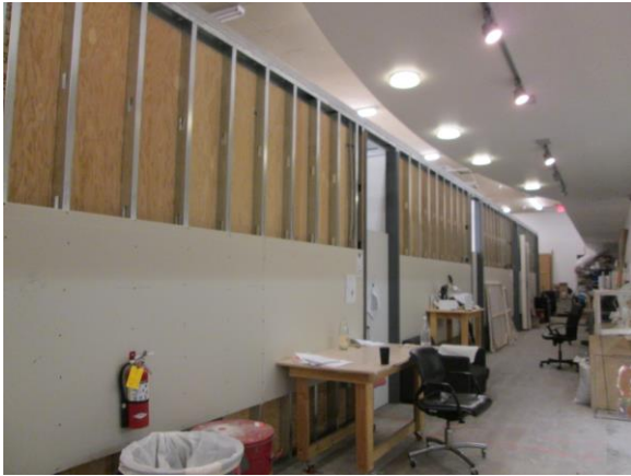
Figure 18: Interior, representative condition. Temporary metal stud partitions (GPA, 2018)
