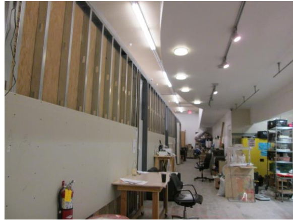
Figure 19: Interior, representative condition. Temporary metal stud partitions (GPA, 2018)
