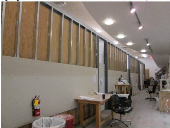
Figure 17: Interior, representative condition. Temporary metal stud partitions (GPA, 2018)
